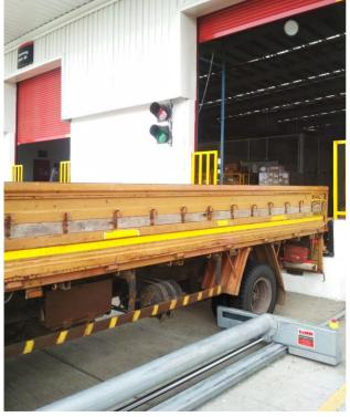
An integral sensor in the wheel block accurately determines the position of the raremost wheel , where upon the wheel block is automatically extended and the wheel is restrained.
